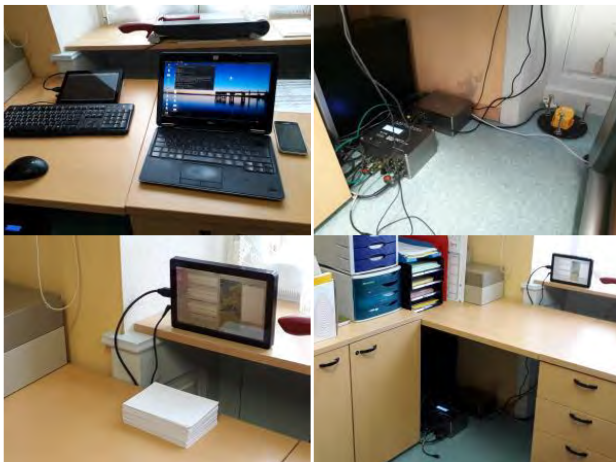
Figure 3 A prototype MP-Wise sensor installed on May the 14th 2018 in the town hall of the village of Keffenach. The sensor was customized by considering the specific fragility model of the building.
